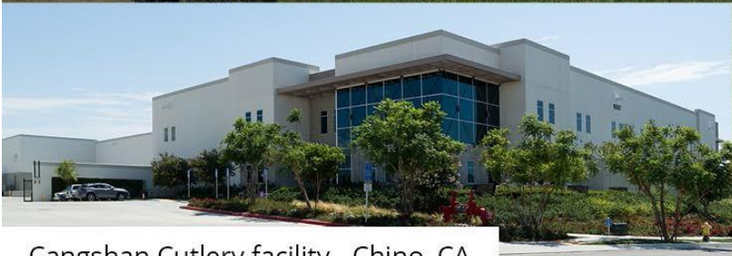
Cangshan Cutlery facility - Chino, CA
